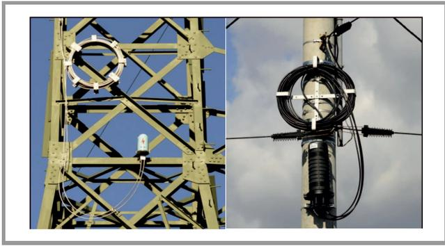
**Fig. 8.** Spare lengths of aerial fiber optic cable accompanying a joint closure box: OPGW on a 400 kV high voltage power line (left) and ADSS on a low voltage line (right).
